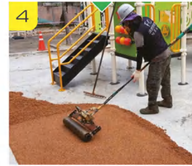
Open after curing
