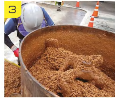
Coated cork chips-binder agitation
